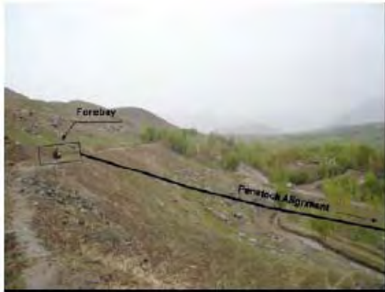
3. Forebay and Initial Penstock Alignment
