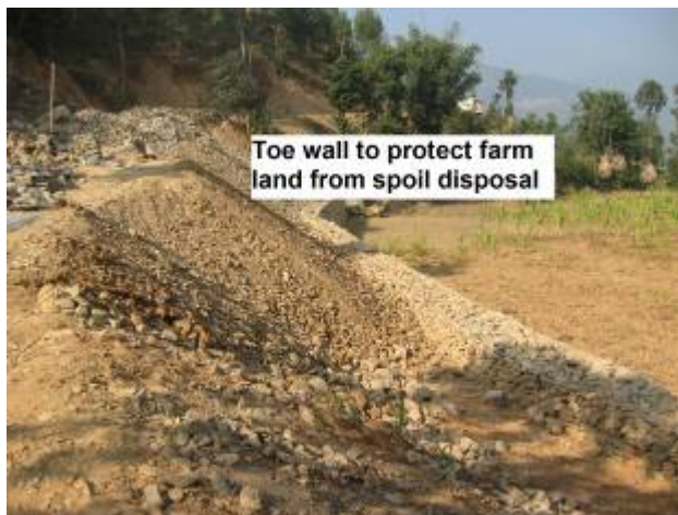
Toe wall constructed at Ch 9+300
