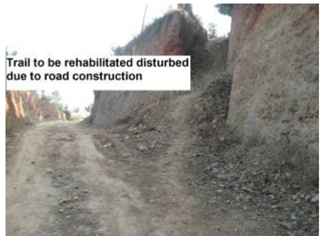
Trail to be rehabilitated at Ch 11+500
