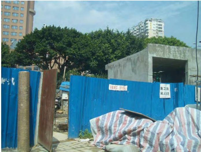
Component A: Yangli Phase II Sewer Networks
