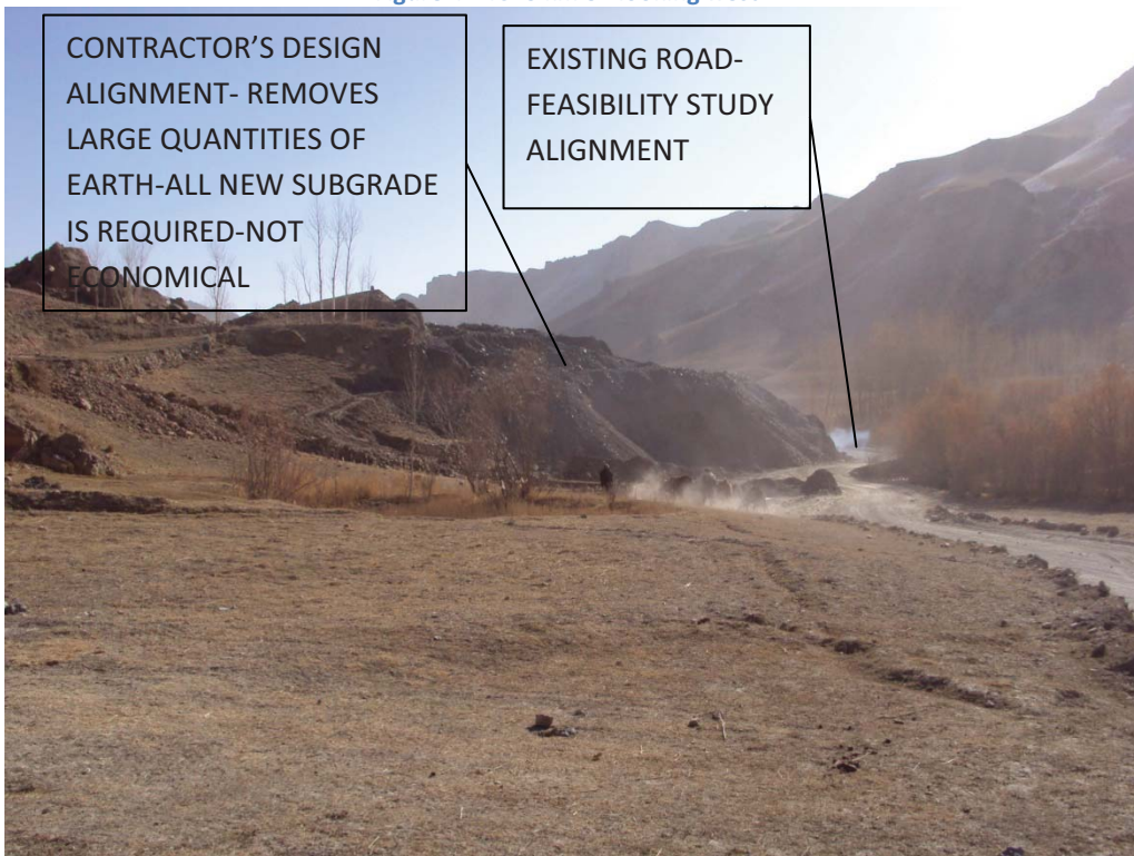
Figure 5 - ICB3 km 81 looking west
