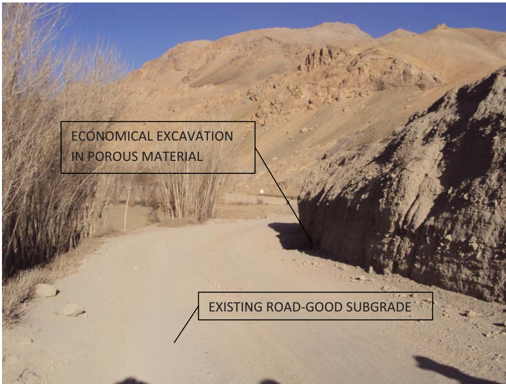
Figure 4 – ICB3 km 81 looking west-
