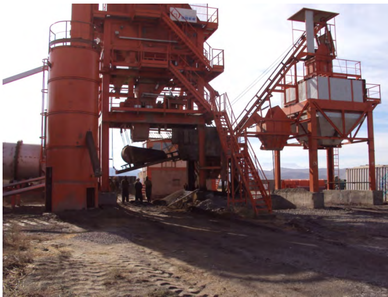
Figure 2 – Asphalt batch plant is idle
