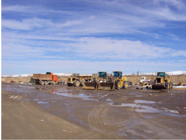
Figure 3 - Idle equipment at the Qasir equipment yard on Thursday, November 26.
