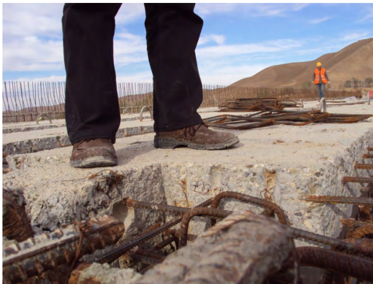
Figure 15 - Girder Positions at Bridge 3
