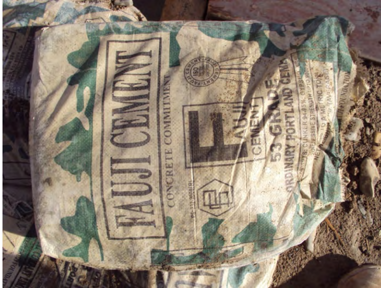
Figure 120 - Cement Bag-Back. Bags do not include the Type I/Type II designation as required by the Engineer.
