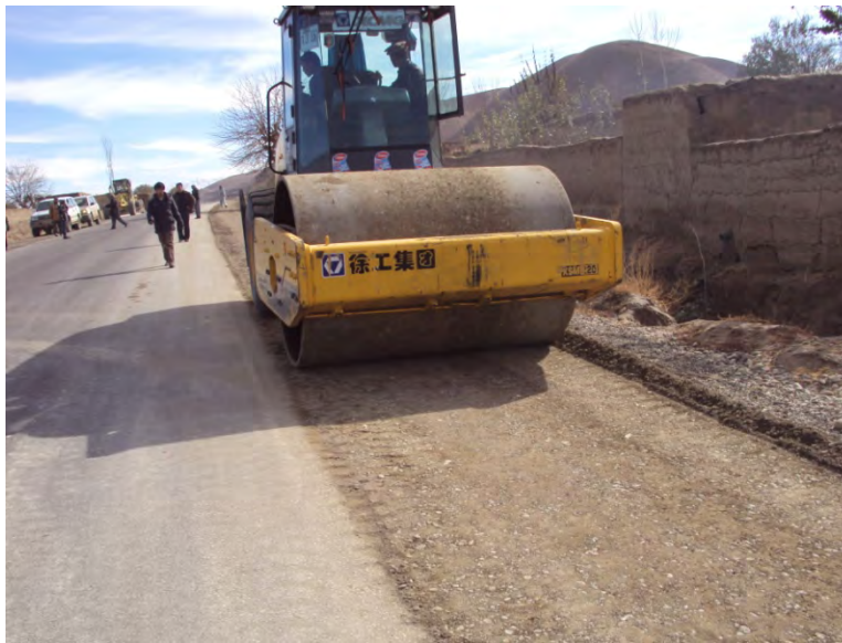
Figure 13 – Hard shoulder compaction
