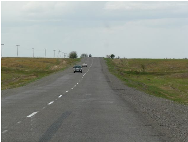
Picture 1. Section 3A, Open Highway
