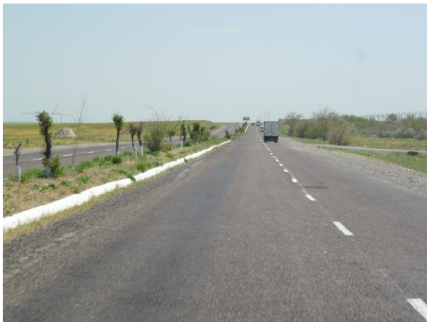
Picture 3. Section 3A, Category 1 segment, near Taraz
