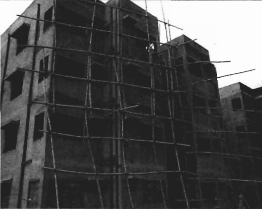
Construction of new flats is going on at Sampamirzanagar
