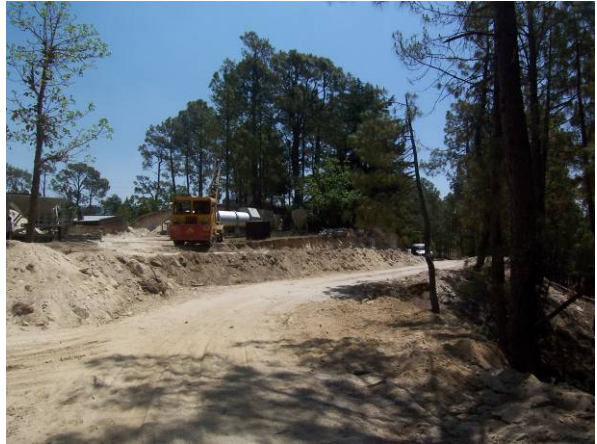
Fig.8: Earth work at construction camp site on Barechhina-Sheraghat Road (Contract VIII)
