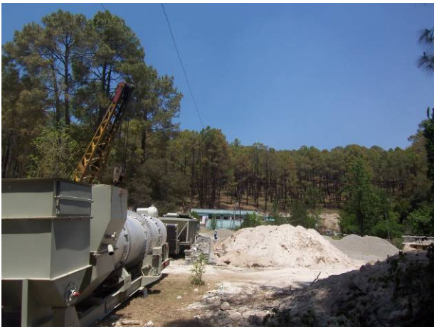
Fig.9: Location of Construction camp at km 95 on Barechhina-Sheraghat Road (Contract VIII)
