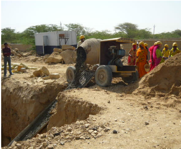
Drain -01 work under progress
