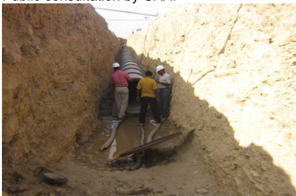
Laying of waste water pipeline
