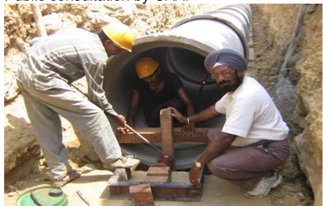
Testing of Pipe
