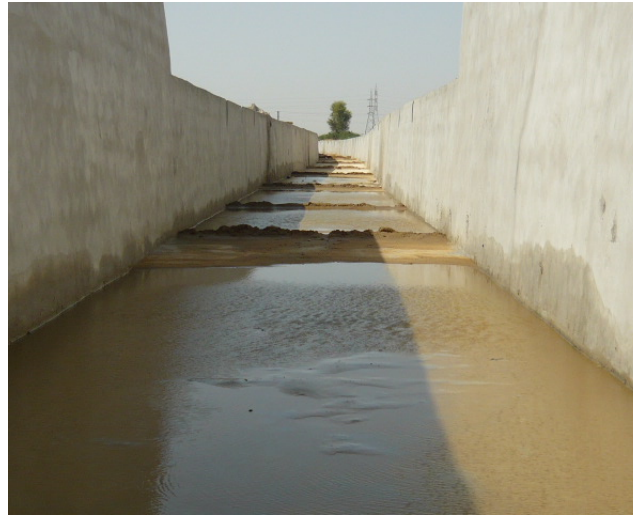
Completed part of drain
