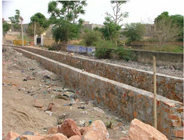
New construction of Drain
