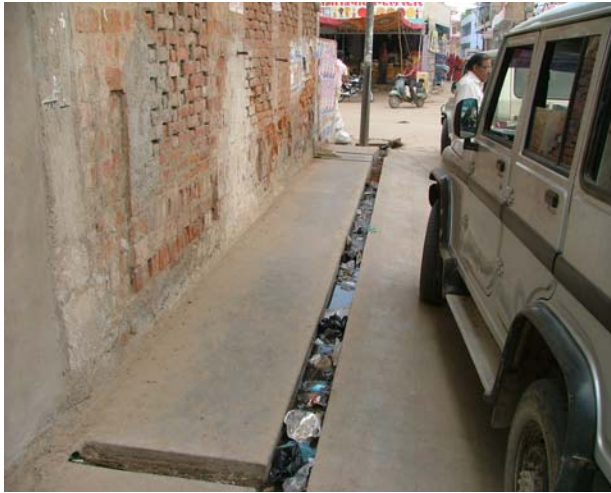
Existing condition of drain
