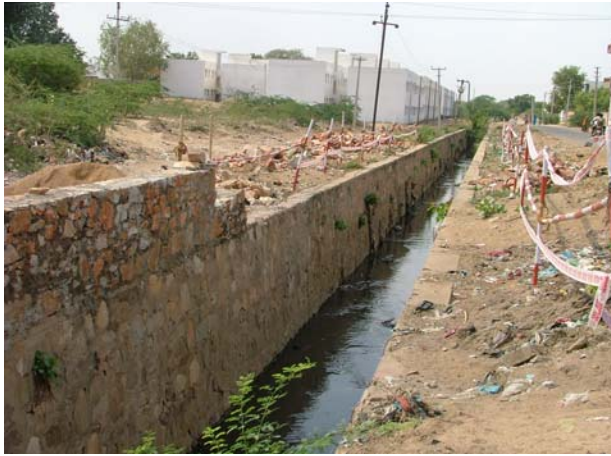
Old and New construction
