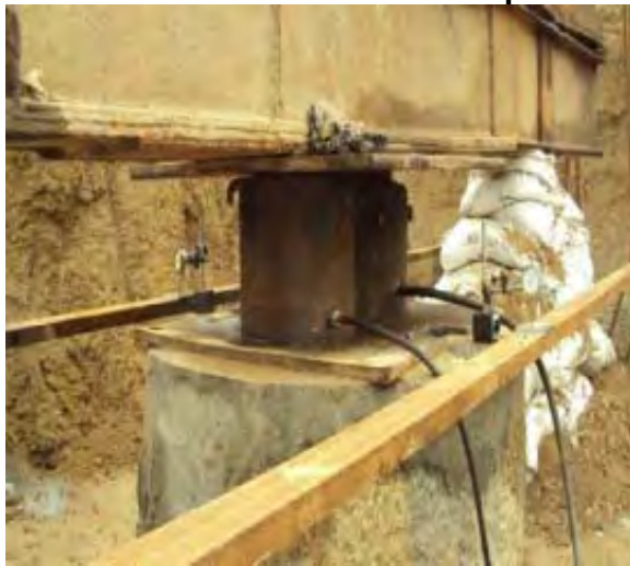
Routine Pile Load Test
