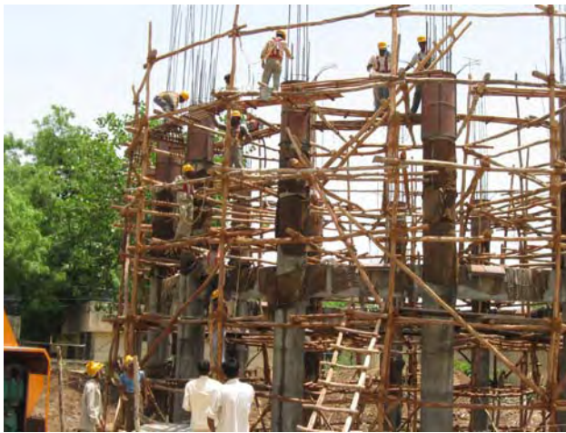
Photo 1: Column casting at TEJ MANDI OHSR for ALW/WS/02- Utilisation of PPE like helmet, safety belt noted
