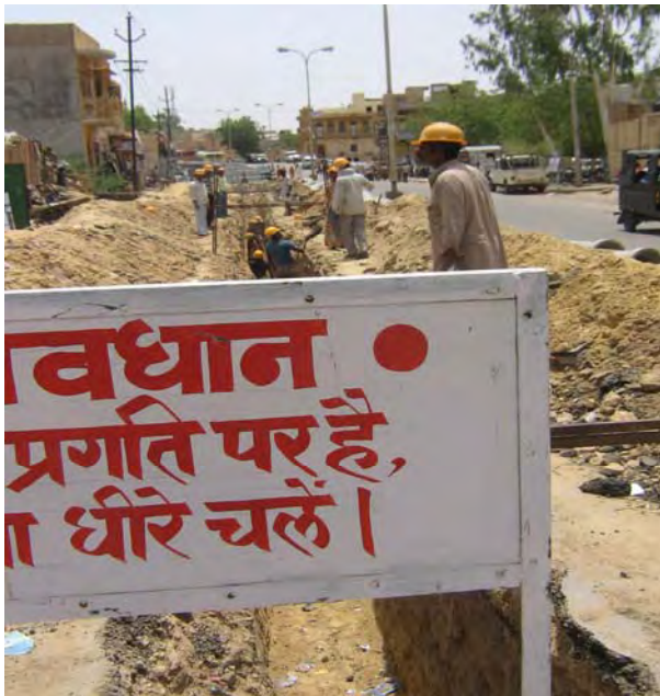
Photo 15: Caution Board – at project site
