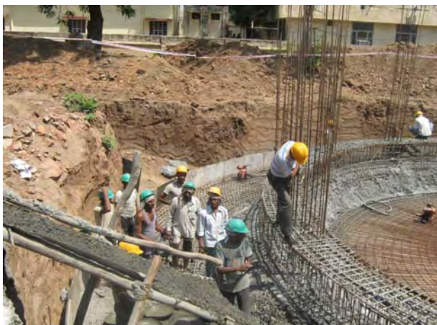
Photo 5: Utilisation of helmet at OHSR site
