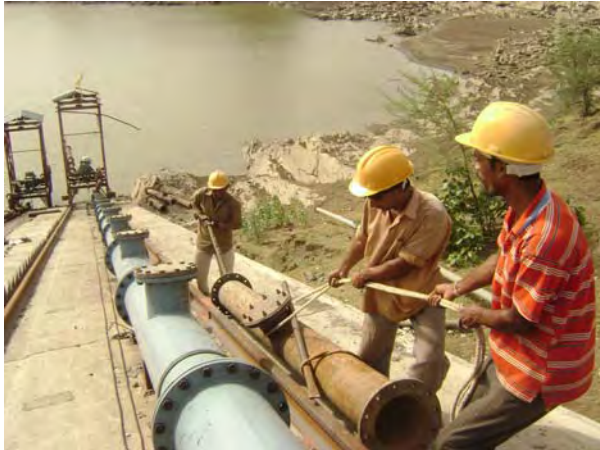
Photo 9: Railing works under progress in Pipaji – ka-Deh, Intake site, Jhalawar
