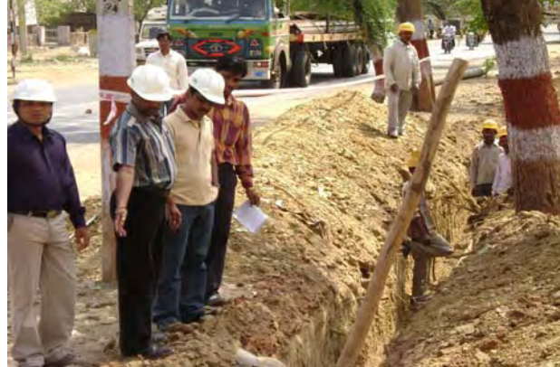
Photo 8: Pipe laying Works Near NH 12- safety ribbon and use of PPE noted
