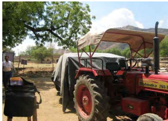
Photo 4: Covered materials during Transportation- Tej Mandi site
