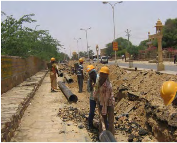
Photo 13: Use of PPE at water supply Package Pipe laying site- Jaisalmer
