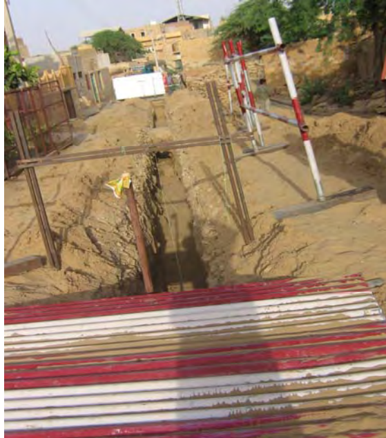
Photo 16: Barricading and movement platform at project site
