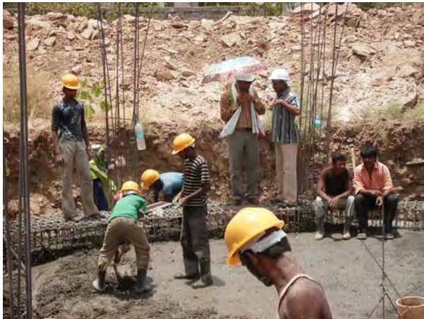
Photo 11: Constructional works under progress at Balaji – ki Chattri ESR - personal safety considered
