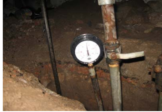
Photo 20: Pipe line testing going on at Alwar
