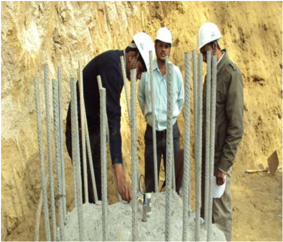
Photo 21: Integrating Testing – Alwar bridge
