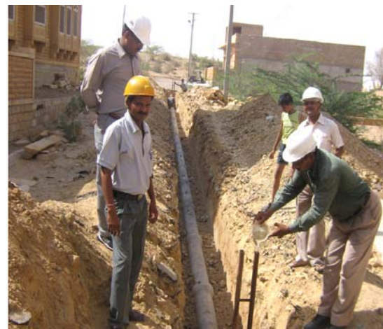
Photo 6: Testing of Sewer line at Jaisalmer
