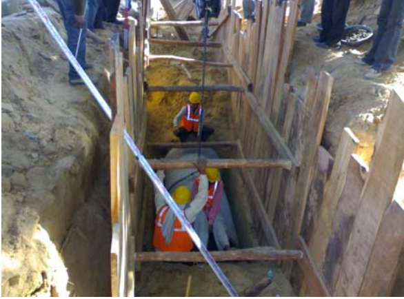
Photo 19: Work under progress for Sikar Sewerage
