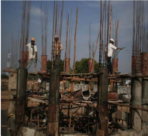
Photo 9: Work in progress at Topkhana ESR at Jhalawar
