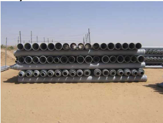
Photo 17: Proper storage of material at Jaisalmer
