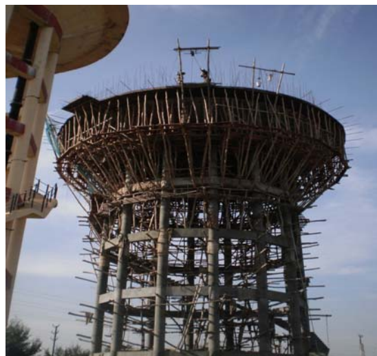
Photo 10: Work is going on at Balaji ki chatri ESR site- Jhalawar
