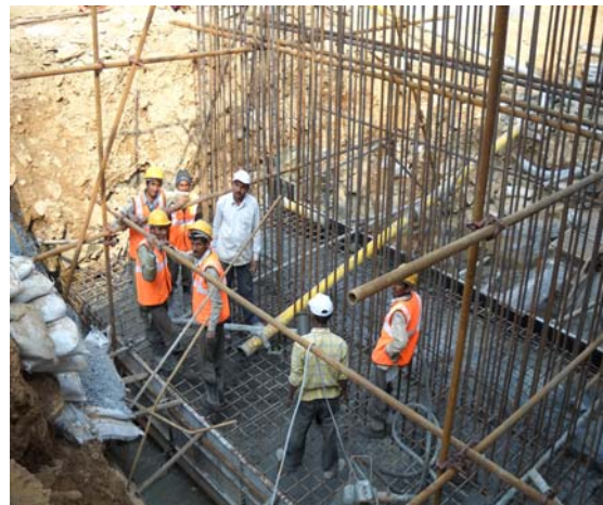
Photo 12: Work in progress at Chittorgarh Bedach bridge- use of PPE noted
