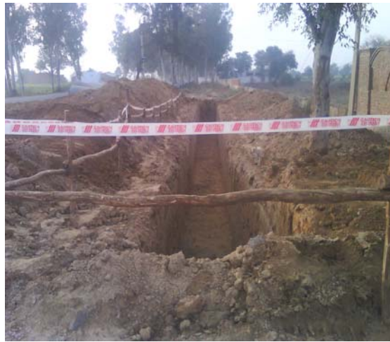
Photo 22: Laying of Pipe Line at Alwar - safety caution tape noted
