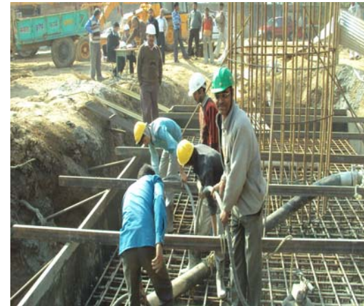
Photo 4: Work is going on at Alwar bridge site
