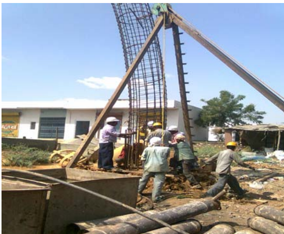
Photo 5: Bridge construction in progress at Sawai Madhopur
