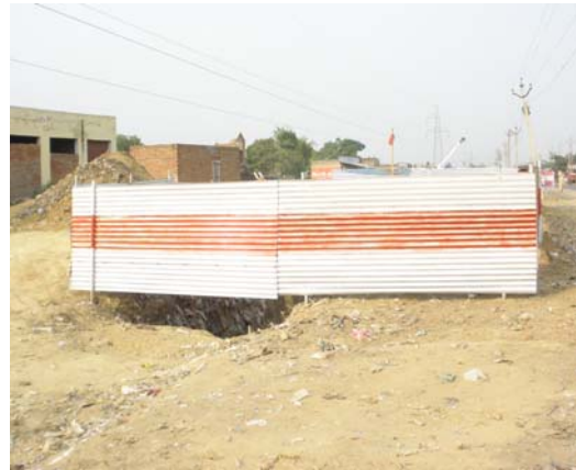
Photo 2: Barricading near excavated area for waste water package at Alwar
