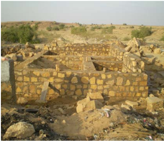
Photo 7: Building construction at landfill site under Jaisalmer
