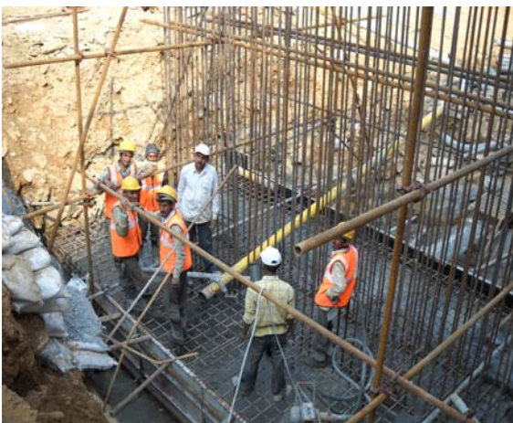
Photo 23: Pier construction at Gambhiri river Bridge at Chittorgarh
