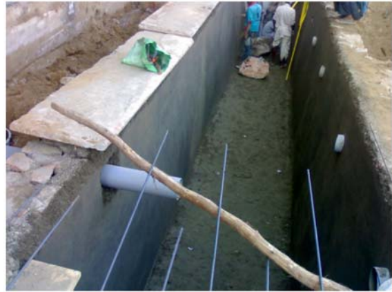
Photo 8: Drainage work under progress at Sikar
