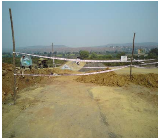
Photo 14: Rising main road crossing in progress at Jhalawar
