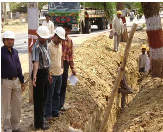
Photo 11: Pipe laying Works Near NH 12 at Jhalawar
