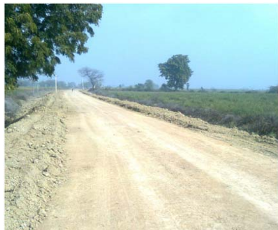
Photo 24: Road diversion work going at baran for construction of bridge
