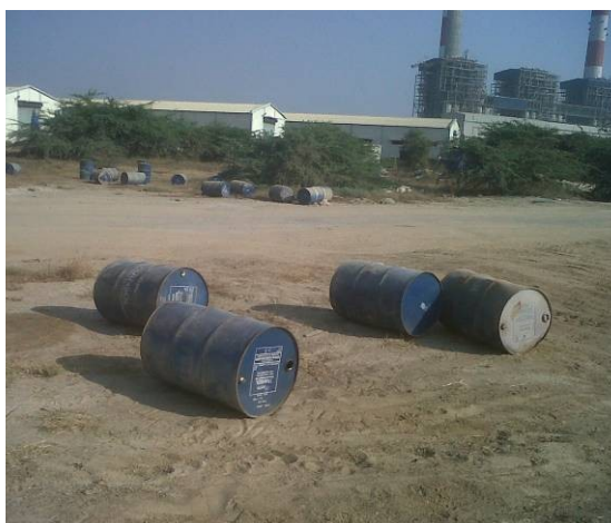
Photo 5: Indiscriminate storage of transformer oil drums
