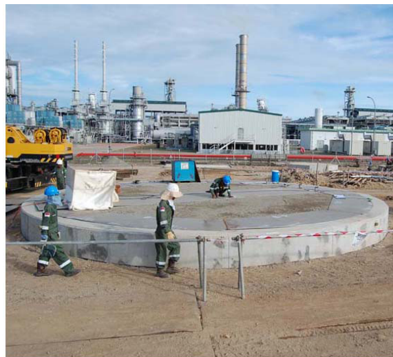
Figure 2. Commence Bottom Plate Erection of Tank TK-34
