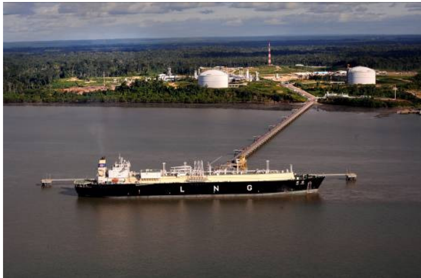
Figure 1. LNG Plant and its Supporting Facilities, with LNG Tanker in the Foreground
