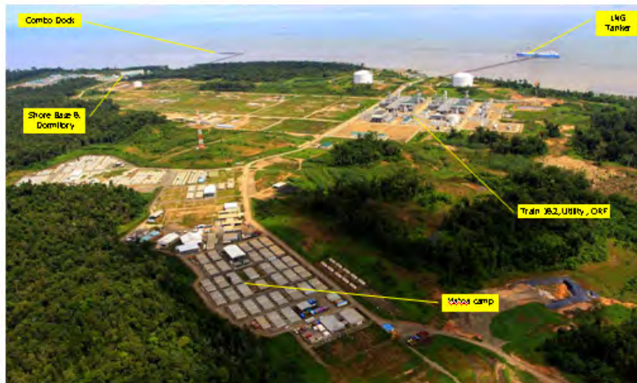
Figure 1. LNG Plant and its Supporting Facilities
