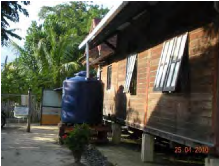
Figure 3 Back-up Water Tank in Tanah Merah Baru
