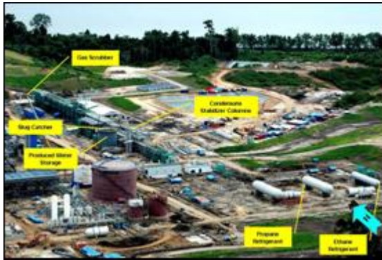
ORF & Refrigerant Storage
