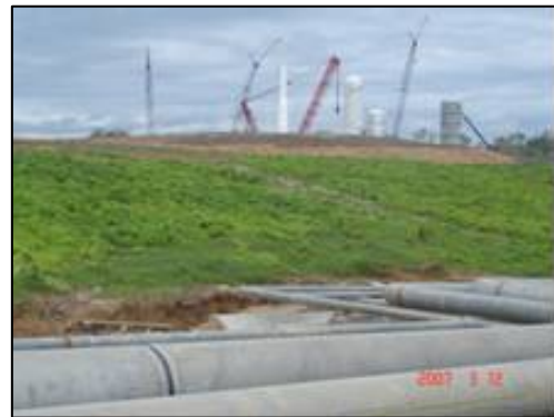
Slope Protection on the Road to Jetty
