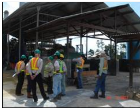
Non Hazardous Waste Incinerators
