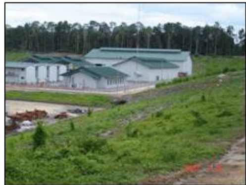
Erosion Control and Land Stabilisation at the Shore Base area
