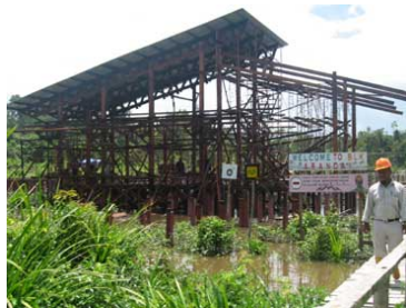
Figure 7: BLK Aranday under Construction
