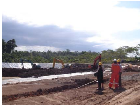
Sanitary Landfill Construction
