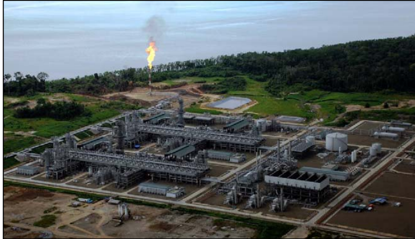
Process Train and Utility
