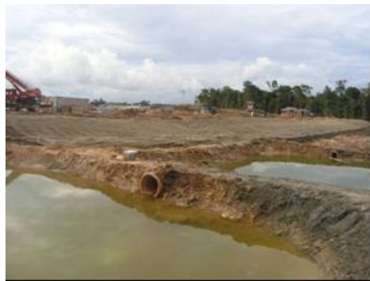
Neutralization pond on GS-30 to Neutralize low pH water
