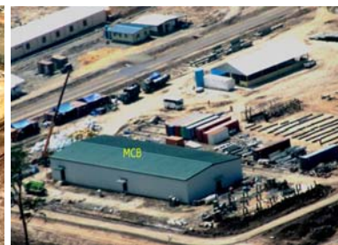
Main Control Room
