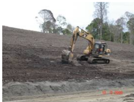
Top Soil Spread on the slope
