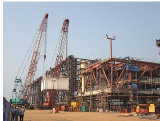
Gunanusa Yard –Technical Building Lifted
