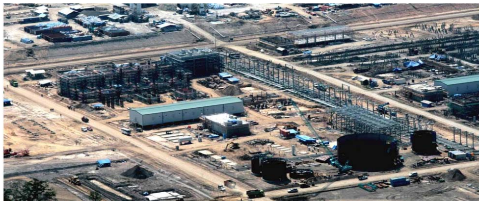
Plant Utility Area
