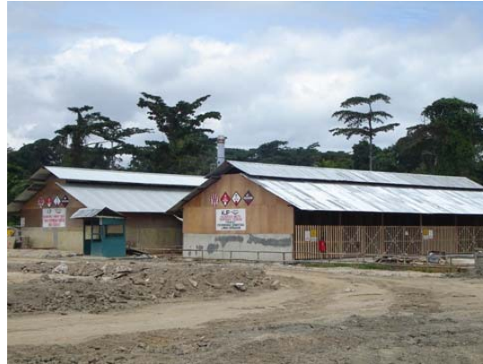
Used oil storage facilities
