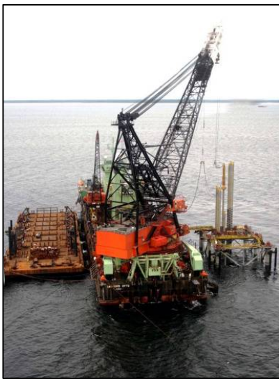
VR-A Piling Installation
