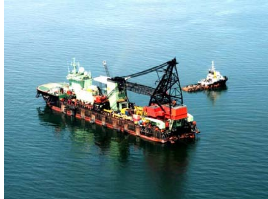
Platform and Pipeline Barge - Castoro-8
