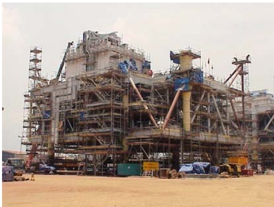
Gunanusa Yard –Deck Fabrication
