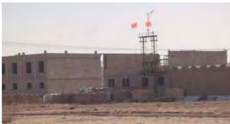
Picture 7: Construction of Centralized Resettlement Site at Dingbian County, Shaanxi Province
