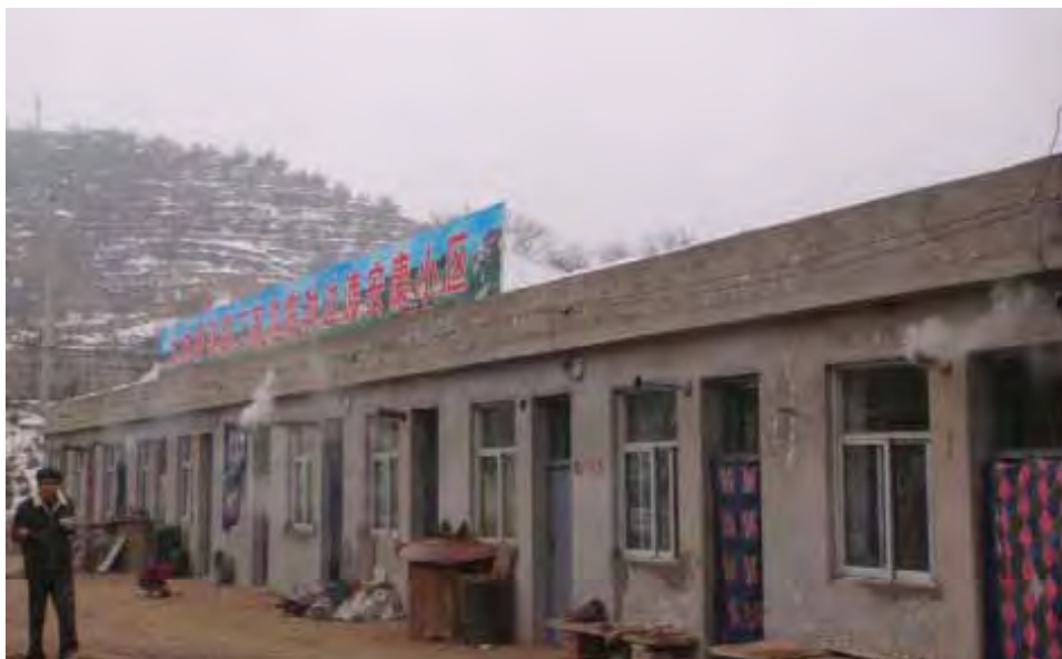
Picture 8: Makeshift Resettlement Site at Suide County, Shaanxi Province
