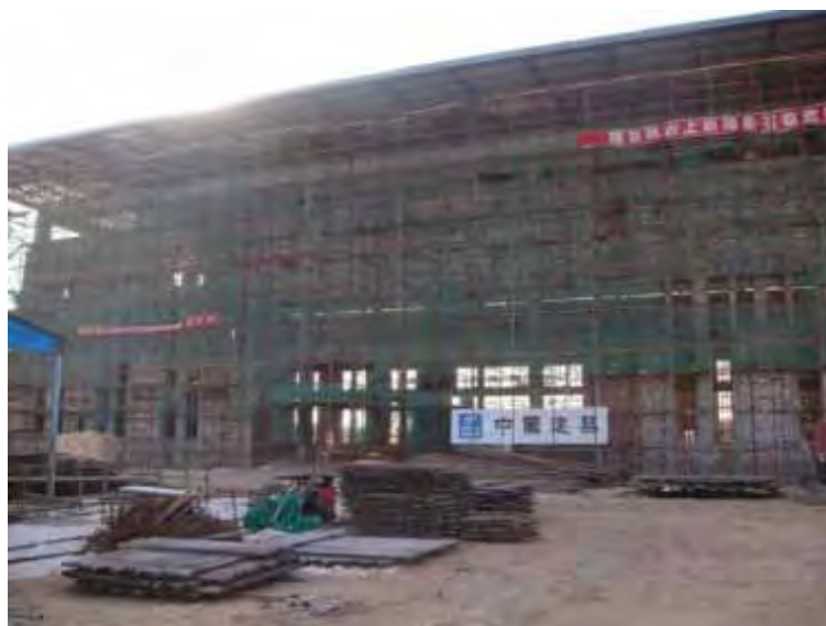
Picture 10: Present Situation of Dingbian Railway Station in Shaanxi Province
