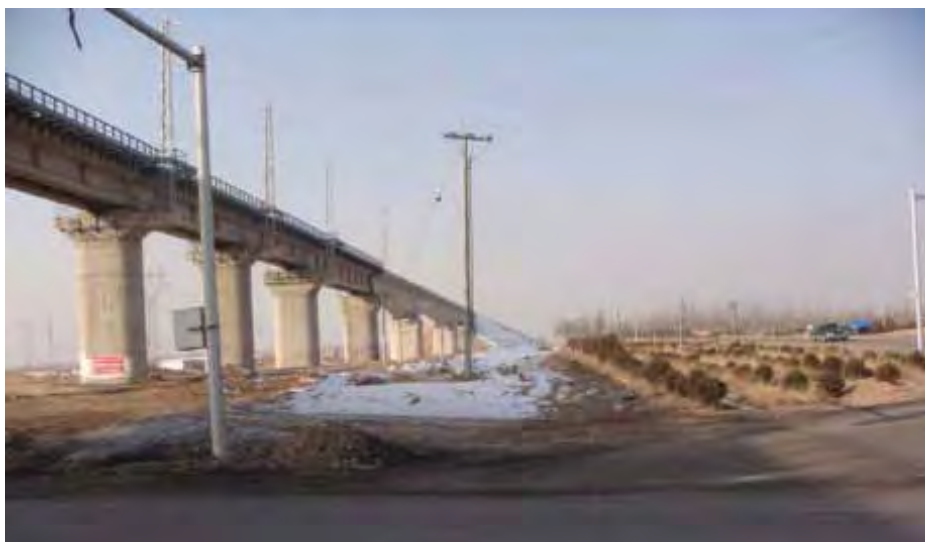
Picture 10: Site of Ningdong Railway Station in Ningxia
