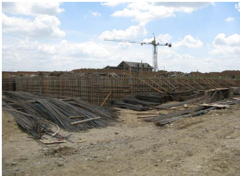
PHOTO3.2- 1 CONSTRUCTION SITE OF SHUANGYANG WTW
