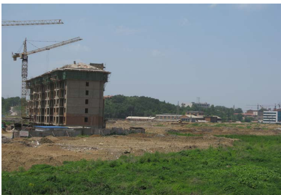
PHOTO3.2-2 DISCARD EARTH YARD OF LIAOYUAN WTW(ORIGINAL LOW BOTTOMLAND)
