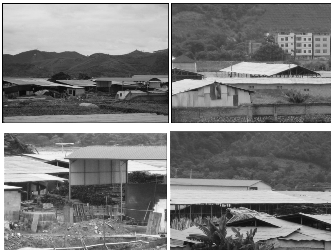
Figure 3 Wood Processing Factory to be Demolished
