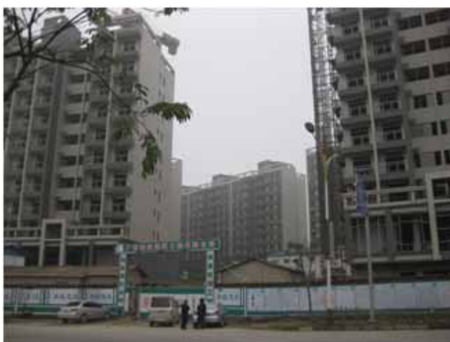
Picture 2-1 Construction site of Fengling New Village
