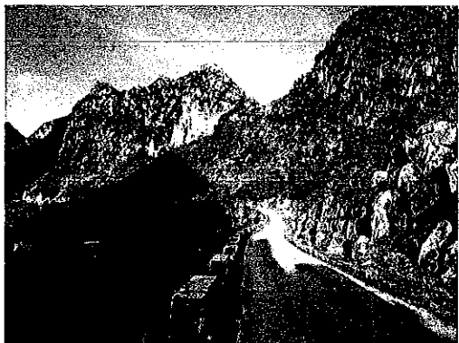
Figure3 Road at Li group, Chadao village, Jingde township, Debao county
