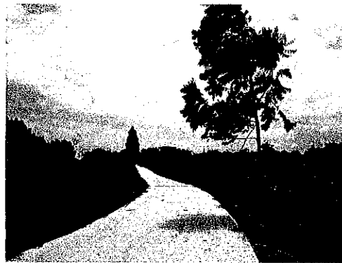
Figure 10 Road at Kuangyuan group, Xiangzhou village, Xiangzhou township, Tiandong county
