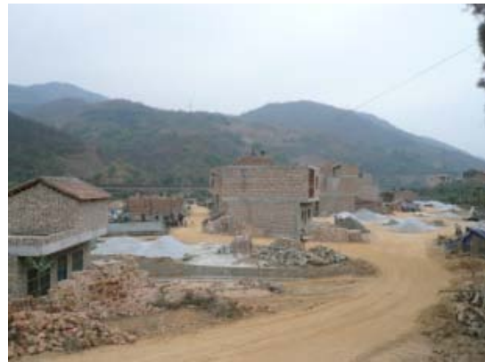
Figure 10. New village under construction at Hongqi group in Hongqi village
