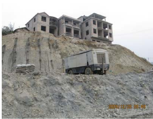
Figure6. New houses reconstruction at Nami landslide
