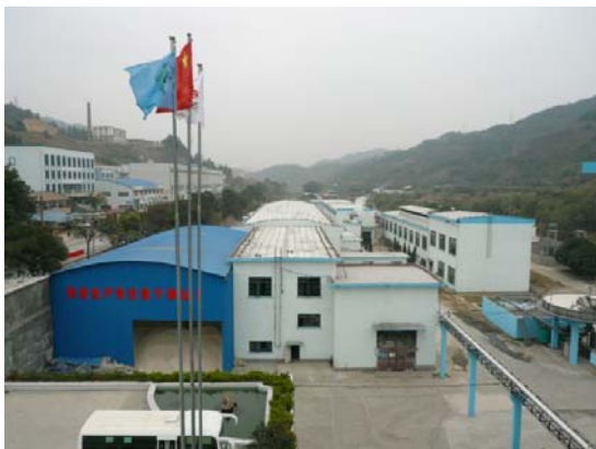
Figure11. New constructed workshop
