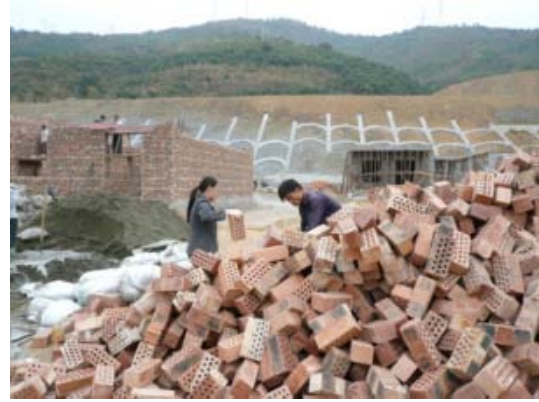
Figure8. Resettled people press on with new house construction
