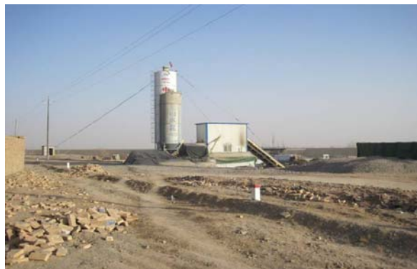
Construction Site Along the Expressway
