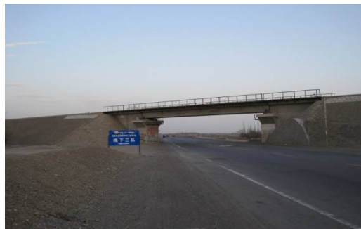
The Overpasses Being Built
