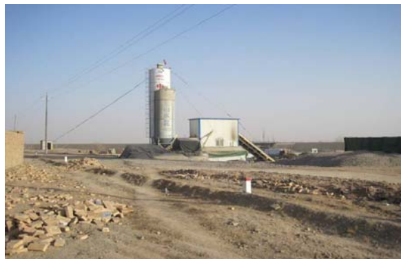
Construction Site Along the Expressway
