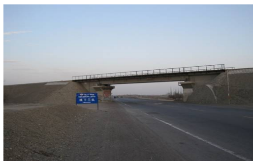
The Overpasses Being Built
