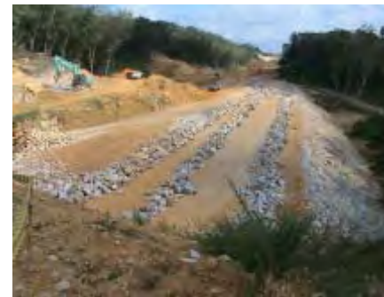
Embankment erosion control measures at Ch. 58+700
