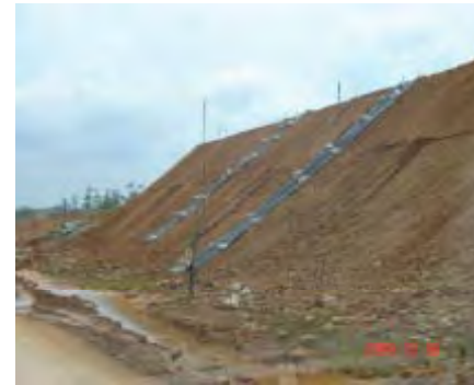
Embankment erosion control measures at Ch. 58+700
