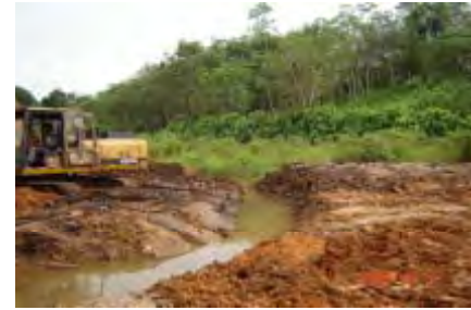
Provision of drainage at disposal site at Ch. 50+500 (RHS)
