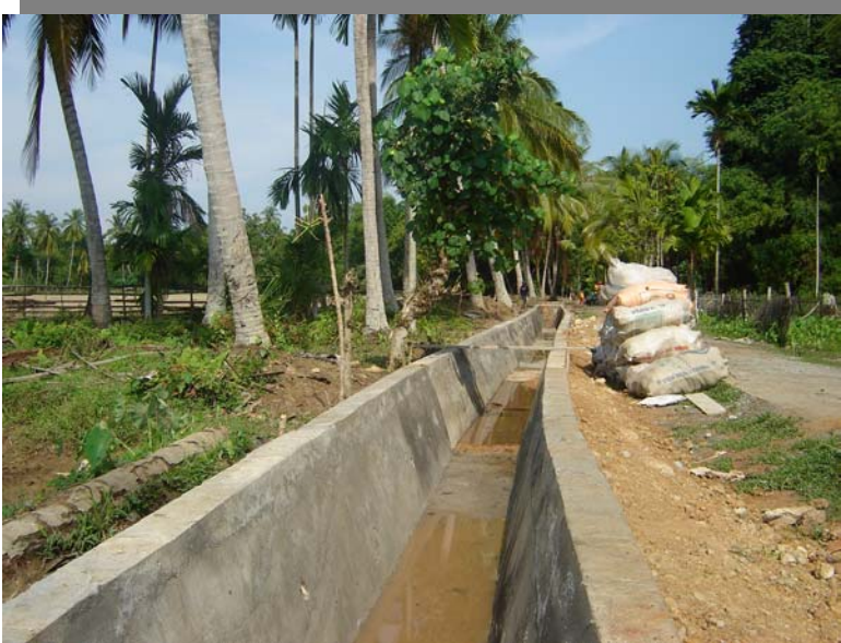
Figure 5: Water User Association (WUAs) are able to construct high quality secondary canals, instead of tertiary ones. (DI. Alue Ubay, Aceh
