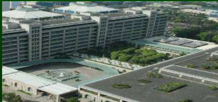
The orientation of the buildings minimizes heat on the east and west facades, the areas exposed to morning and afternoon sun
